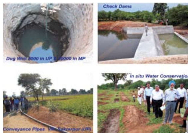
Fig.1. Rainwater harvesting, efficient conveyance, in situ conservation and recharging of wells in Bundelkhand region.
